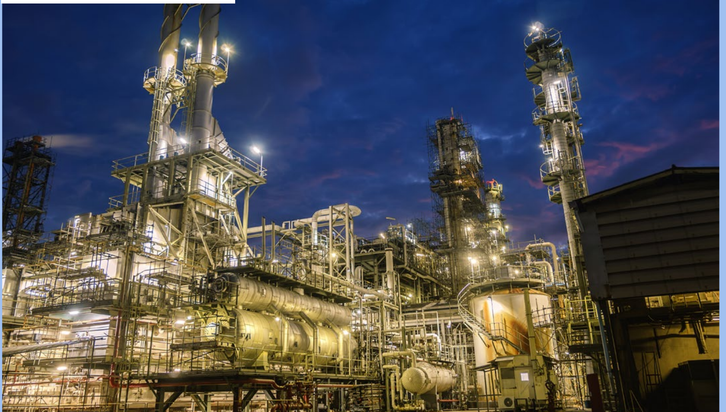
Petrochemical Plant Shutdown Maintenance
